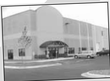
Ford Motor distribution center building in Menomonie, Wisconsin. Ford and GM both located parts distribution centers in western Wisconsin in the past year.
