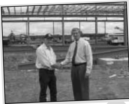
Fred Riermann (left), President of American Structural Metals, and Forward's Ken McAdams in front of the American Structural Metals construction site in Somerset, Wisconsin.
